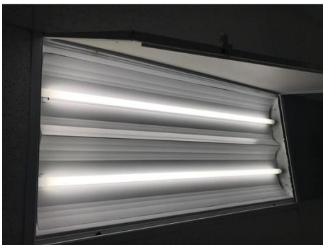
2x4 troffers in the main area with 2 T5 lamps each
