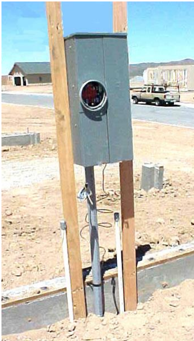
Figure 2 Surface Mount Panel w/ 2"x4" Stud Framing
