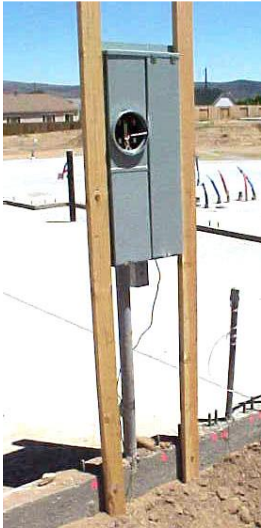
Figure 5 Semiflush Panel Mounting Using 2"x4" Stud Framing
