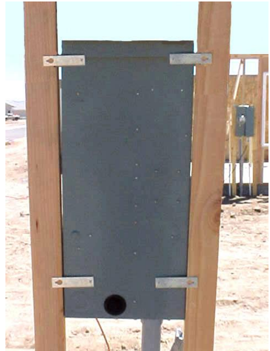
Figure 3 Panel Back Showing Swing Out Mounting Brackets Attached To 2"x4" Stud Framing
